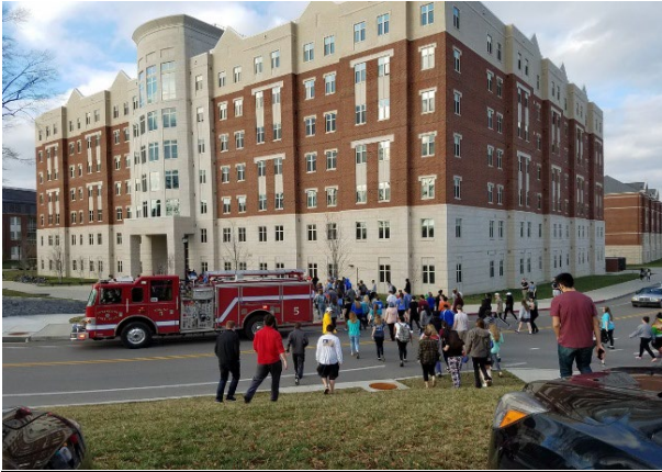
Unannounced scheduled fire drill at resident halls
